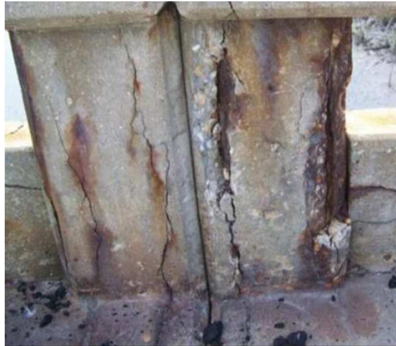
Harriett's Bluff Road at Deep Creek Bridge
