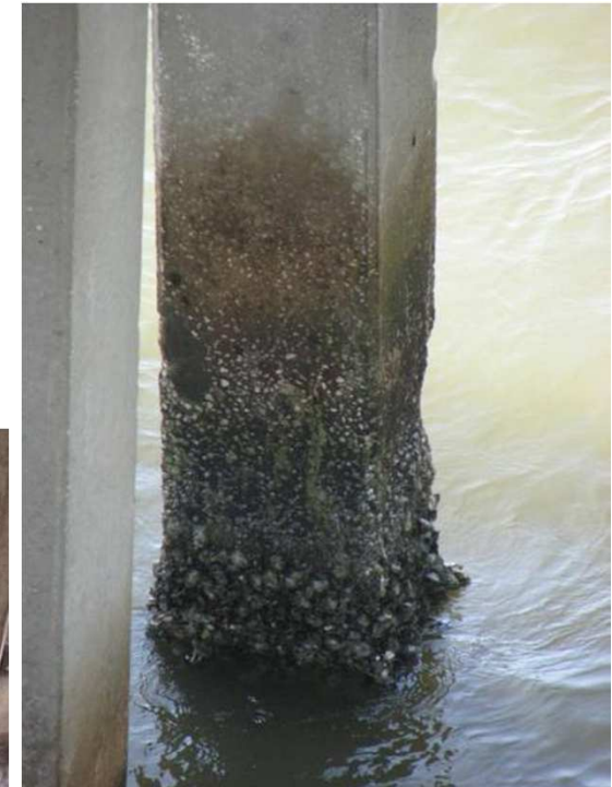
Island Expressway at Wilmington River Bridge
